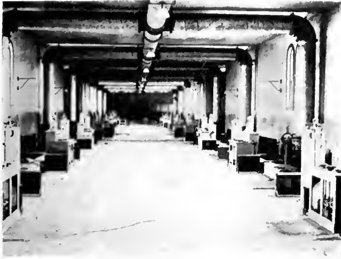
Fig. 6—Completed Prefilter Gallery.
